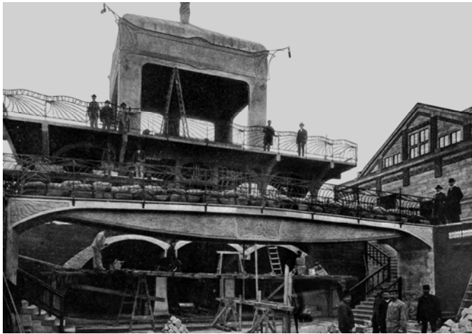
Figure 7: Test load on the bridge by Rudolf Wolle company at the Dresden City Exhibition 1903 (Bastine 1903, plate XVIII).
